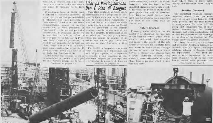
NEW VACUUM Still stack rises some 180 feet above ground. Project, which began in November, is scheduled for completion this July. Bell Caribbean is handling bulk of construction work on the unit. Otis Sidelotom and Earl Sharp are in charge.
